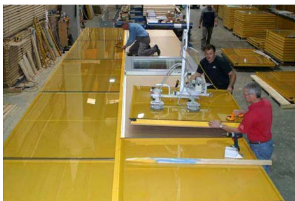
▲ Factory assembling of a large, prefabricated façade module (Austria).
