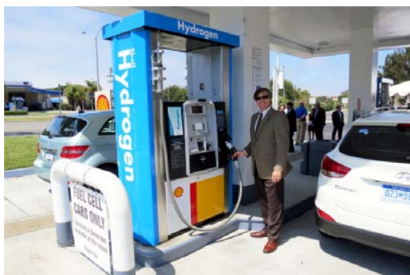
▲ This on-site, small-scale reformer provides hydrogen produced from natural gas to 10-12 customers per day (Long Beach, California).
